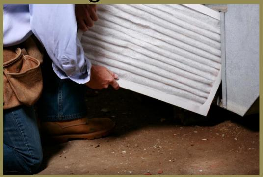
When the filter of your air conditioner cooling system has choked with dust and dirt the performance of air conditioner is reduced by 20%.
